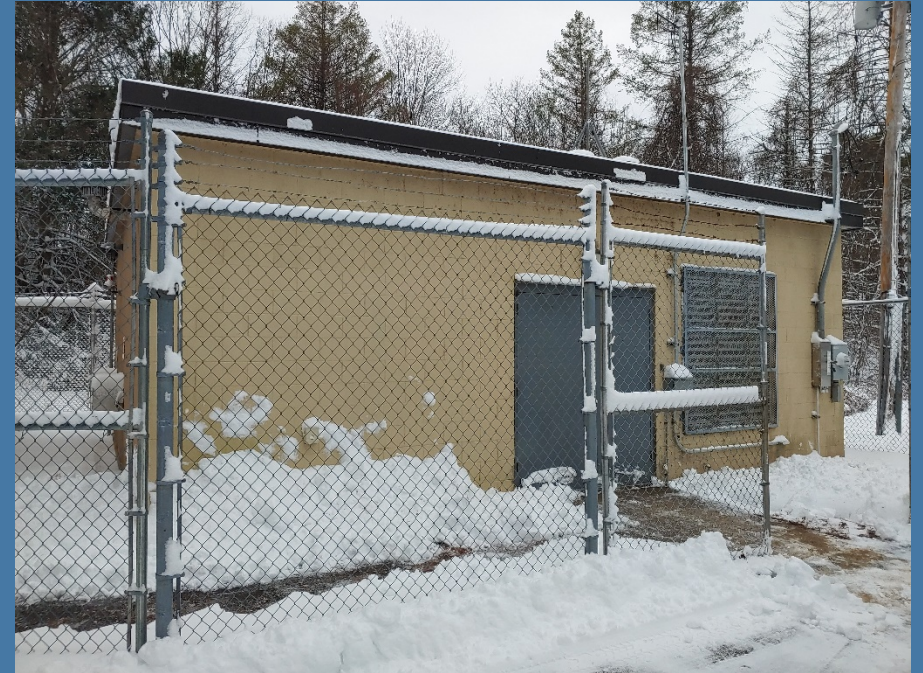
Treatment Facility #3 Building Exterior
