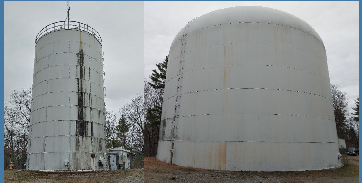
Knuckup Hill Storage Tanks (250,000 gallon left and 1,500,000 gallon right)
