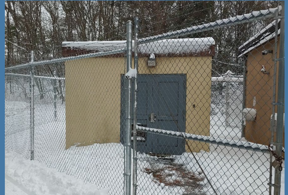
Well 3 Building Exterior
