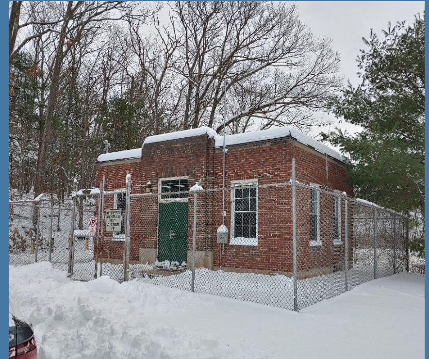
Well 2 Building Exterior
